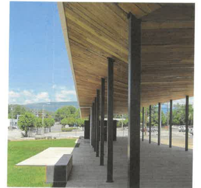
OPEN AIR PAVILION
