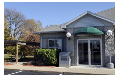
SPENCER TOWNSHIP BRANCH 14960 Meddler Ave. Gowen, MI 49326
