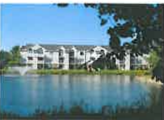
Windmill Lakes 2900 Millpond Drive, West Holland, MI 49424 No. of Units: 402
